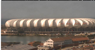
Nelson Mandela Bay Stadium - Port Elizabeth
